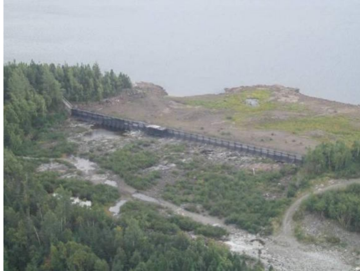
Figure 2 - Rattling Lake Overflow Spillway
